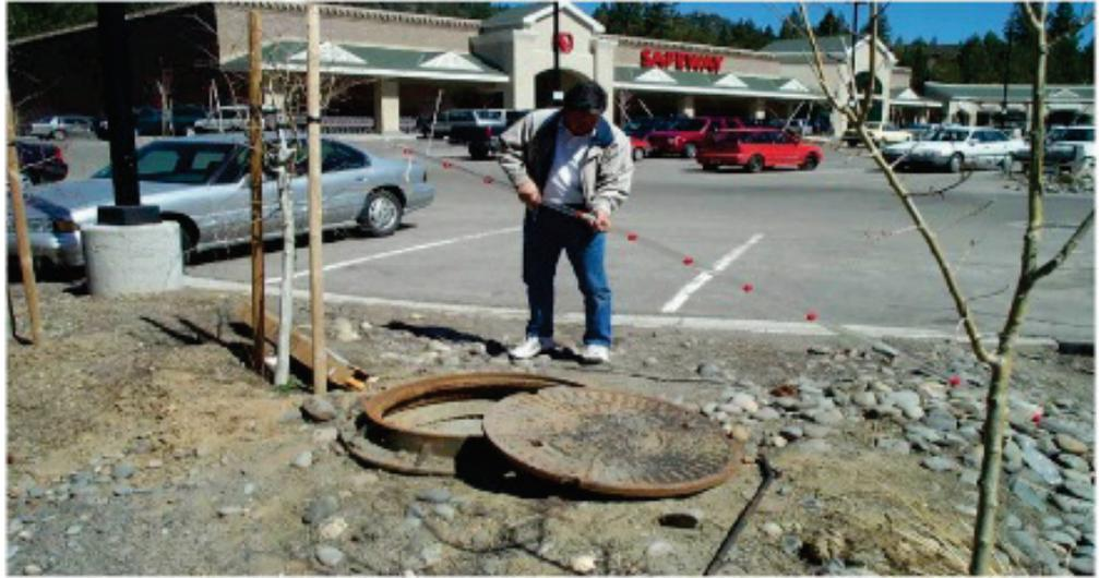
*Inspection of a baffle vault to determine the depth of sediment accumulation and whether oil/grease absorbent pads need replacement.*
