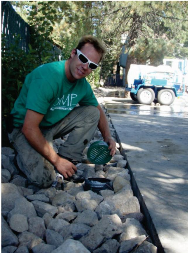
*Contractor showing an inspection port open to visually assess for sediment accumulation in a rock infiltration trench.*
