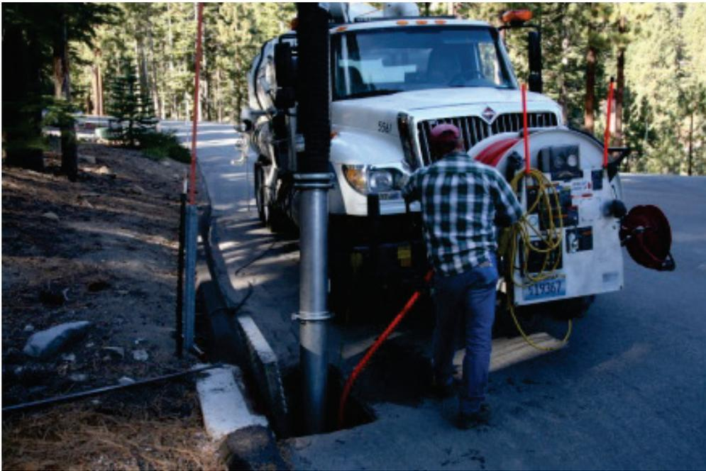
*Vactor equipment removes sediment and other debris out of a drop inlet, preventing re-suspension of materials into the storm drain during the next storm event.*
